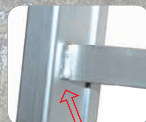
Additional welding on the rung back
