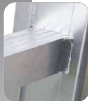
Stile/rung connection through crimping and additional welding
